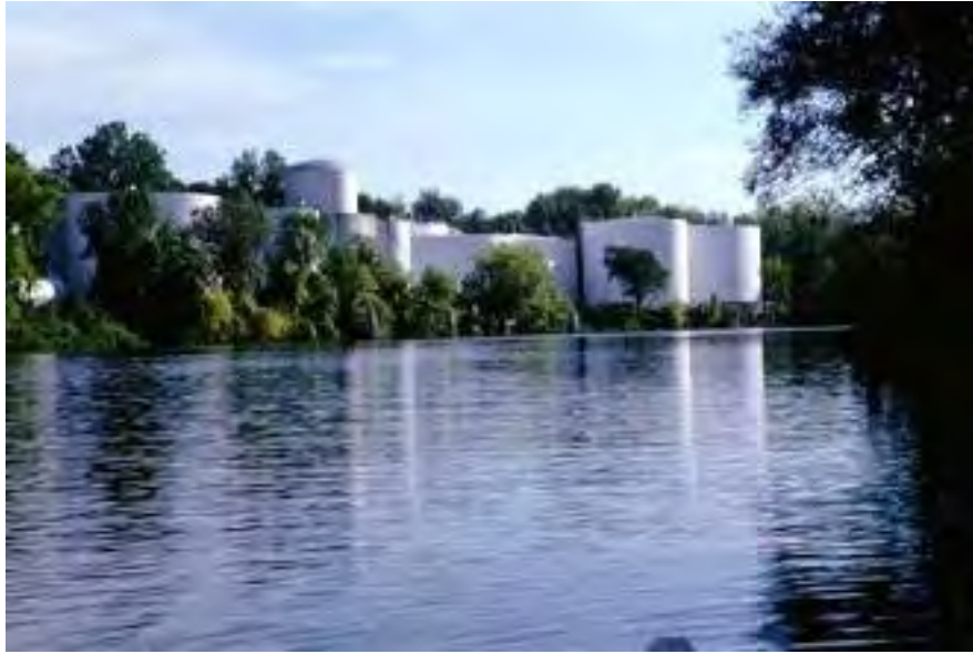
Figure E5-12: Example of Petroleum Fuel Storage near a Water Body
