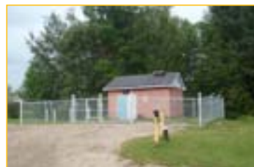
Improved security around a municipal well
